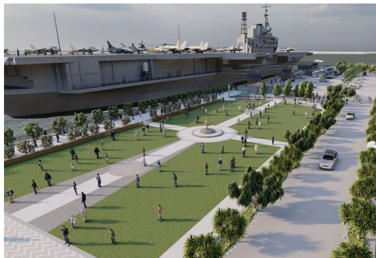
The USS Midway Museum and Port of San Diego made a commitment in 2004 to one day develop a park on Navy Pier. After many years of negotiations and planning, the California Coastal Commission's approval in February gives us the development permit required to start the process of building the park, your park – Freedom Park at Navy Pier.
