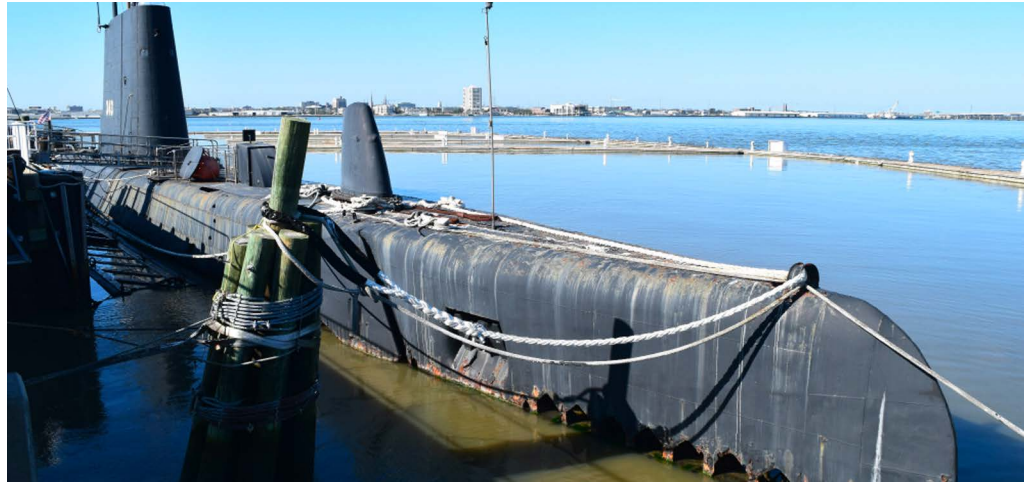
Maintenance staff at Patriots Point found a leak in the main ballast tank of the Clamagore submarine. (FILE/GAVIN MCINT YRE/STAFF)
