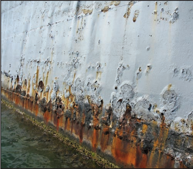
Above: The visible corrosion along the waterline of the ship. Photo by Les Callow.
