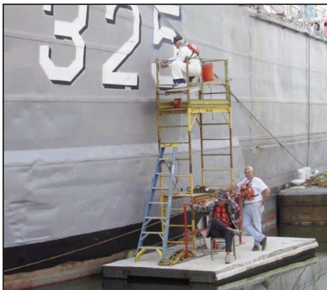
Above: ET Perry Ballinger taking a break from Radio Central to re-paint the 8 ft. tall Port Bow Numbers, assisted by Bill Rockey and Bob Chick, ballast specialists.
