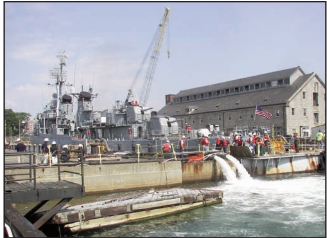
Above: Water is pumped out of Dry Dock No. 1. Photo by Steve Briand.
