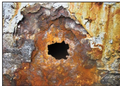
Above: Several holes were found on the forward starboard hull near the water line. Corrosion occurred from the outside, as indicated by the layers. Photo by Les Callow.
