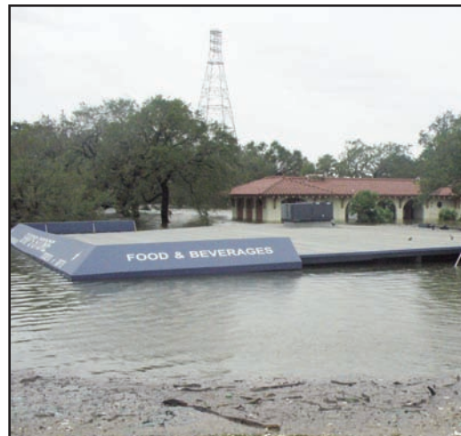
Above: The roof of the Gift Shop/Visitor Center barely breaks above the water following Hurricane Ike.
