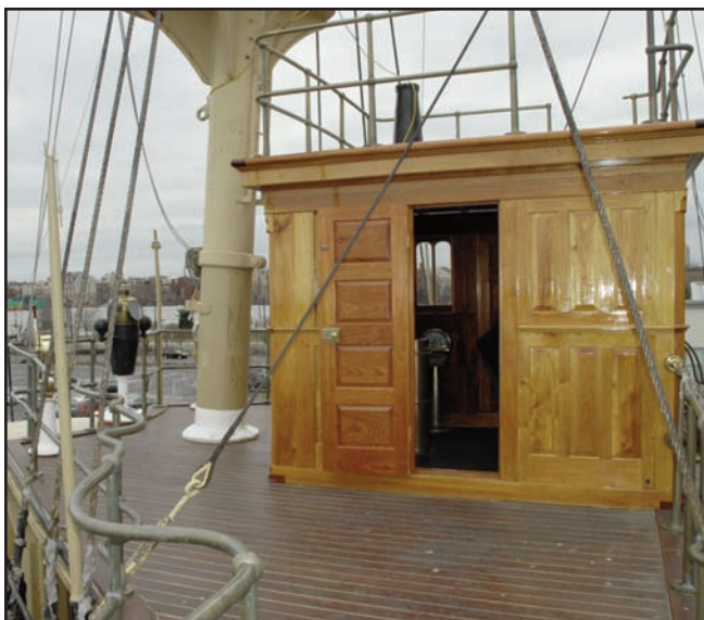
Above: The newly rebuilt pilot house and bridge deck.
