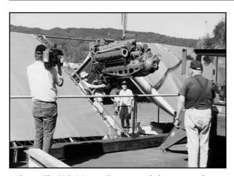
Above: The U.S. Marine Corps provided a crane to lower PT 658's Packard engines into her engine room. All three engines were in place within three hours. Photo courtesy Save the PT Boat, Inc.
